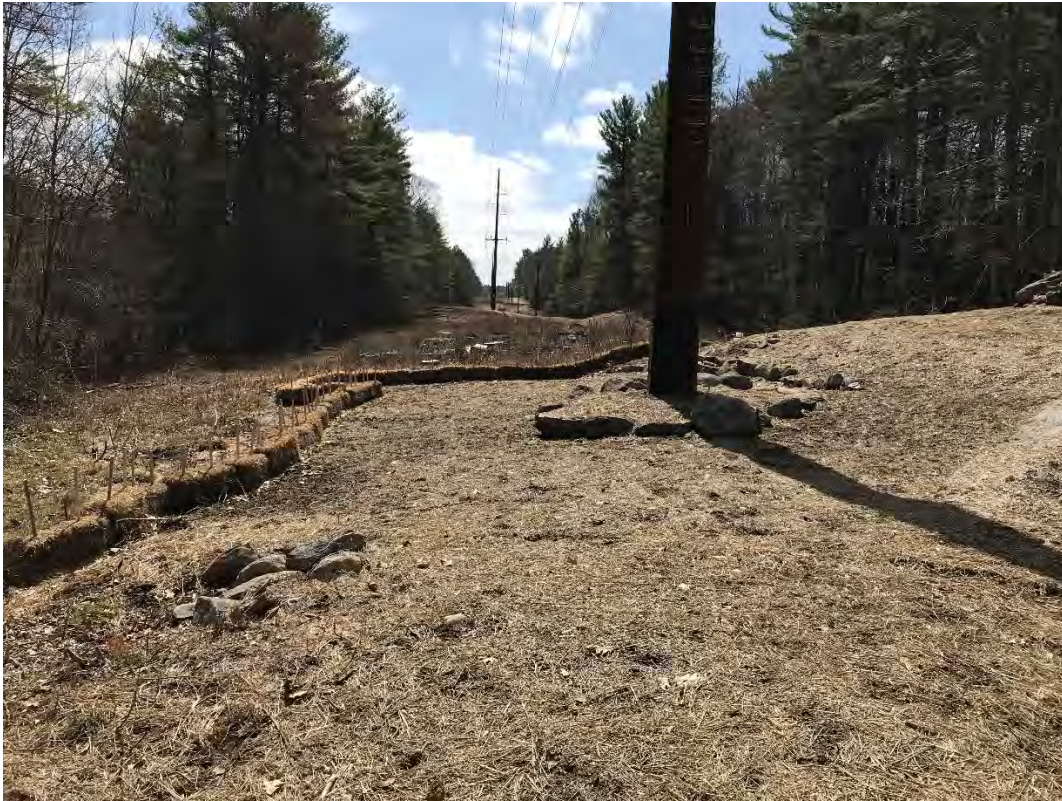
Fig 5: Str. 89 work area. Viewing southeast. (04-14-21)
