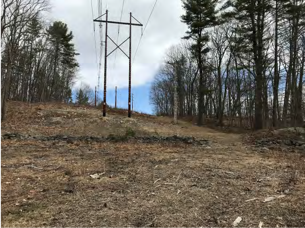
Fig 15: Slope leading up to Str. 57 work area. Viewing northeast. (04-14-21)
