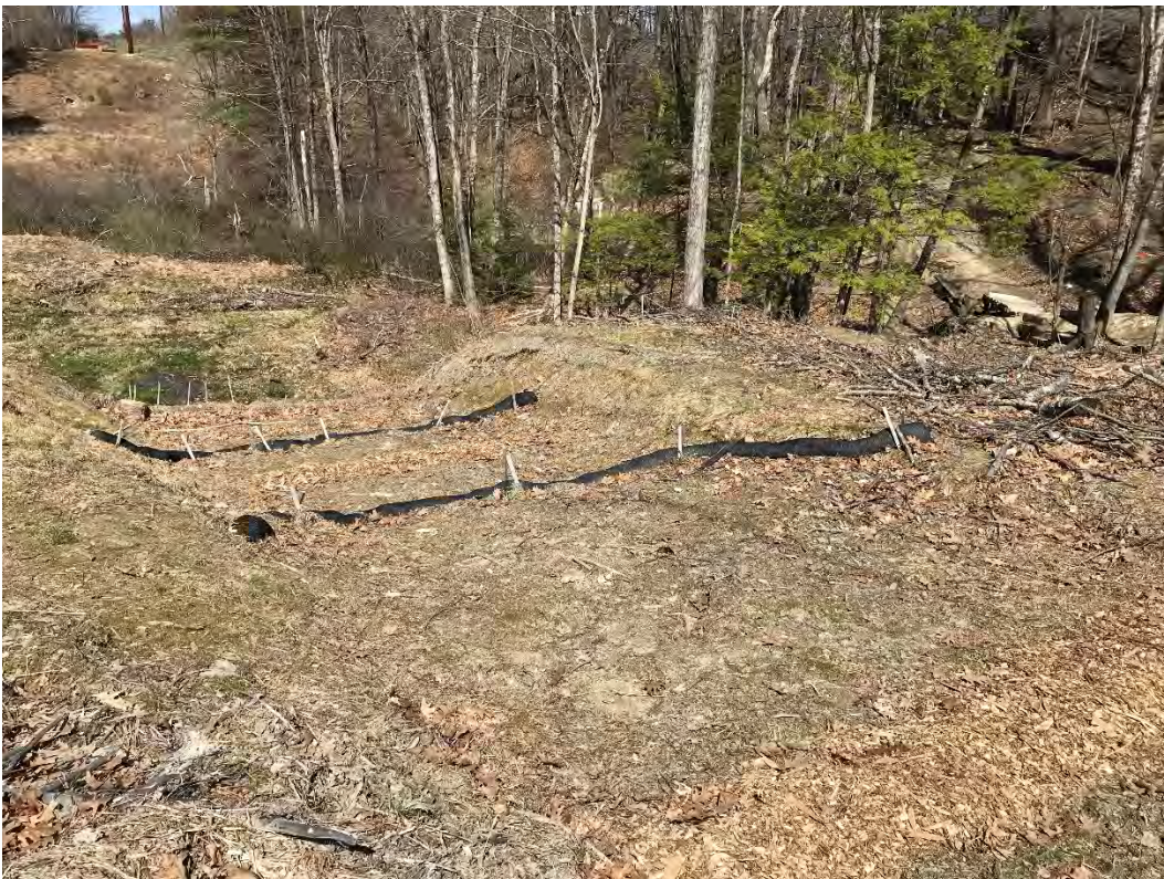
Fig 8: Lower portion of slope between Strs. 28 and 29. Viewing northeast. (04-14-21)
